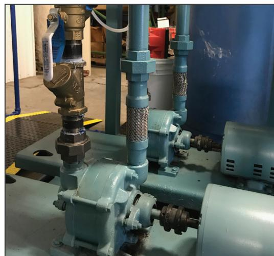
*Pumps that sit idle during the summer months can bind up - check for proper operation*
