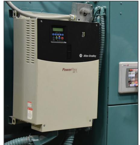
*Variable Speed Drives enable a system to operate only as needed*
